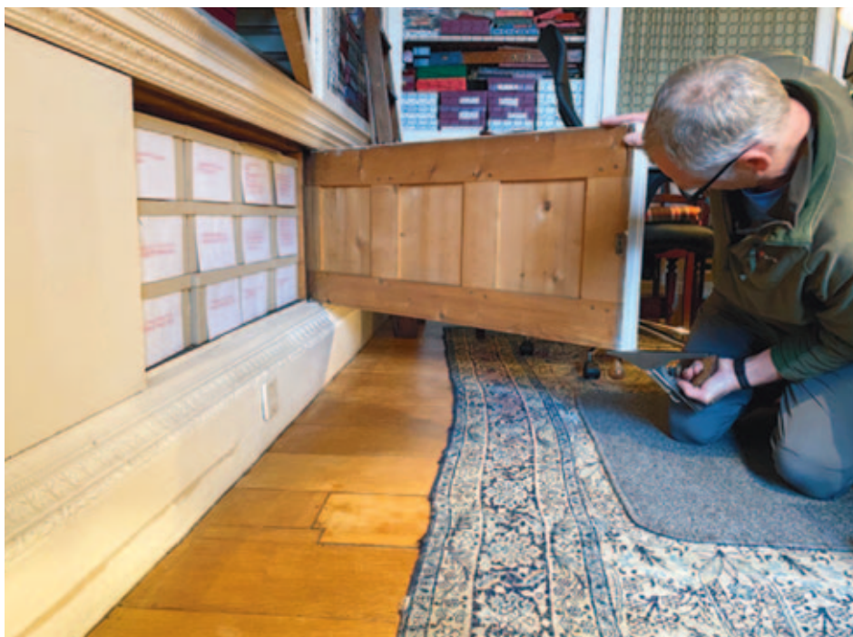
Planing the underside of a door to ease function. Although the hinges are in good condition, some wear means removing material to allow the door to close.
